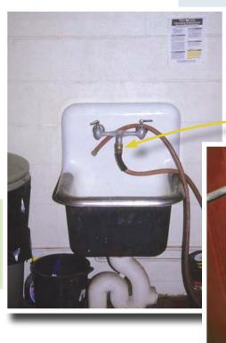
These are examples of inexpensive backflow devices attached to indoor and outdoor faucets.
