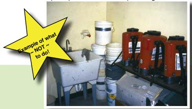
The pipe beneath the sink (right) is disconnected so that drainage is contained in a bucket. It is important to dispose of the bucket contents appropriately.
