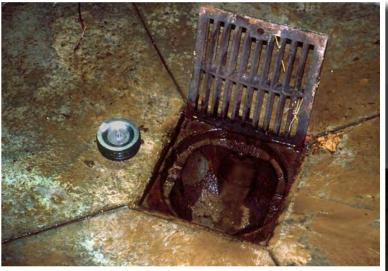
Expansion plug used to seal drain
