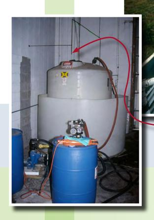
The water pipe in each example is suspended in mid air, leaving an air gap between it and the fill tank.
