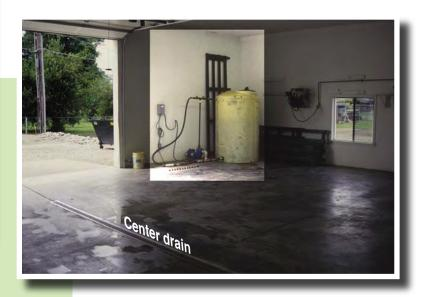
A lawn care company designed their floor to slope toward a center drain (above) which can be emptied into a holding tank in the back of the shop.
