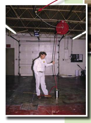
This is a backflow device to prevent siphoning of spray mixture into the well.
