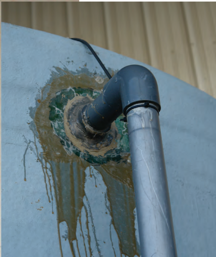
(Left) A sloppy tank repair job. (Right) This tank was properly ground, repaired, and repainted.
