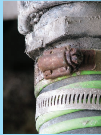
Two clamps (below) provide additional protection inexpensively. Throughout the season, make sure worm gear and T-bolt clamps are properly tightened.
