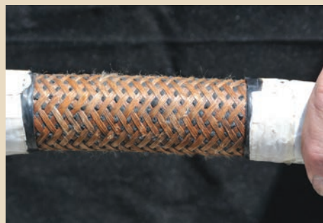
4. Second layer of reinforcing fibers.
